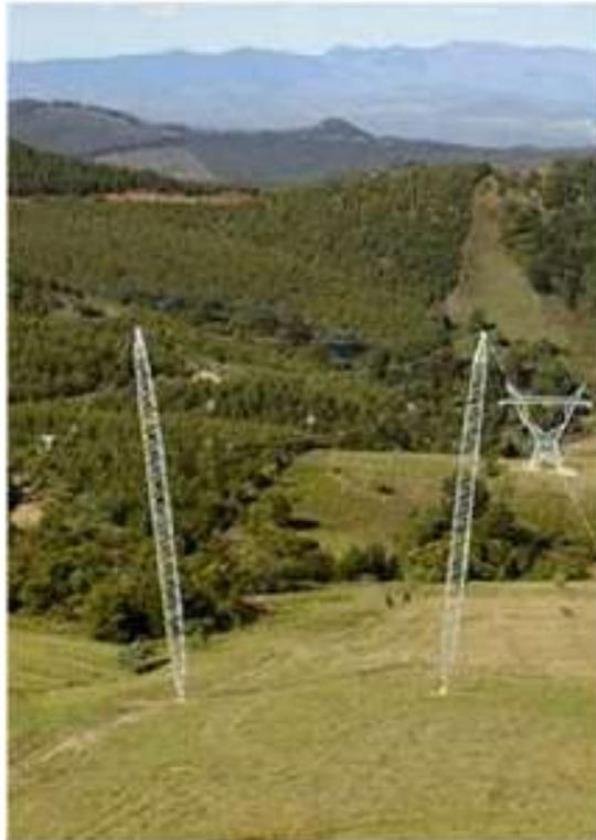
**Figure A-2: Tower Type 524 (Cross Rope).**
