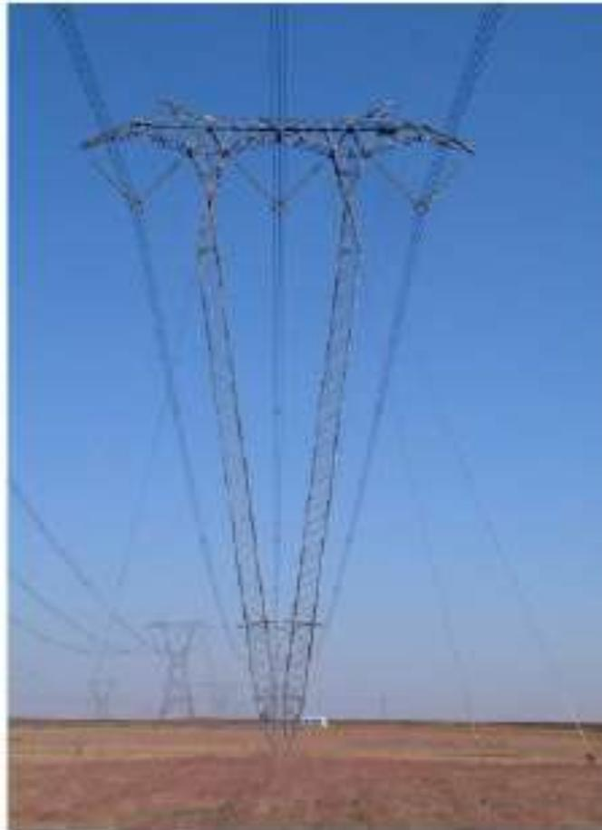
**Figure A-5:** Tower Type 520B (Guyed V).
